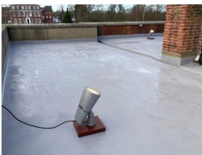
South & West Floodlights setout out on the new roof surface
